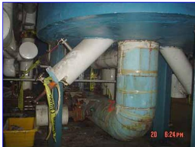
1994 Refrigeration Valves & Systems Corporation Ammonia Vertical Recirculator- 5 ft. dia. x 10 ft. 8 in. H. S/N: 94279. Nat'l Bd: 6718. MAWP: 250 psi @ 300°F. MDMT: -40°F @ 100 psi. Inlets: (1) 10 in. dia. port (suction in), (1) 2 in. dia. port (makeup liquid), (1) 3 in. dia. port (liquid feed). Outlets: (1) 8 in. dia. port (suction out), (2) 3/4 in. dia. ports (vents), (1) 6 in. dia. port (pump suction). Overall dimensions: 7 ft. 2 in. L x 6 ft. 6-1/2 in. W x 13 ft. 7-1/2 in. H.
