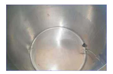
DCI model number code 82 - F - 28940 - A. Was built for a Type A Food Application. This jacketed tank has 1 1/2" inlet/outlet connections for steam and the factory has it rated at 150psi at 100F. It has a heating surface of 22 square foot with 15 on the sides and 7 on the bottom.
