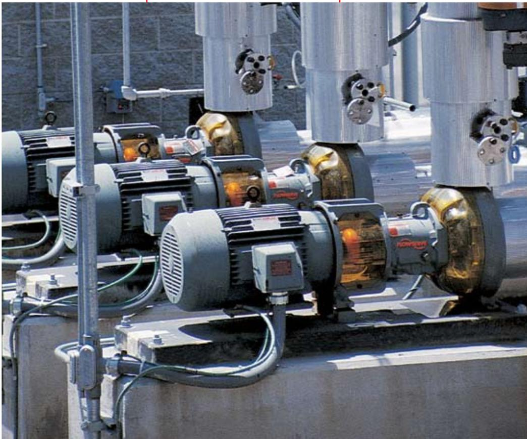
**SealSentry** family of seal chambers features unique flow modifiers (FM) designed to extend mechanical seal life and increase pump reliability.
