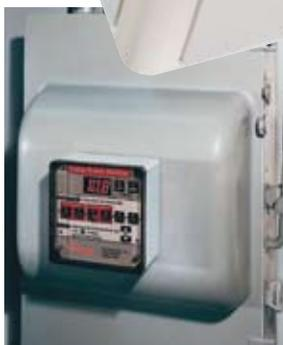
**The KW941 Power Monitor** is easy to install on new or existing pump installations. All connections and controls are located at motor starter electrical enclosure as shown. Costly instrumentation wiring to the pump is eliminated
